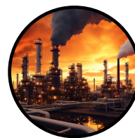
Industrial Waste-Heat Recovery
